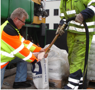
Ejector filling of bead tank
