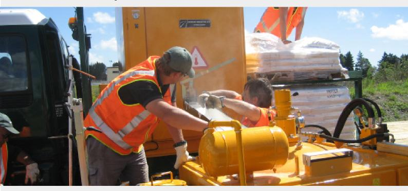
Borum thermoplastic preheaters are melting, heating and mixing the thermoplastic material making it ready for application via the road marking machine. They are provided either as a directly heated (D) or indirectly heated (ID).
